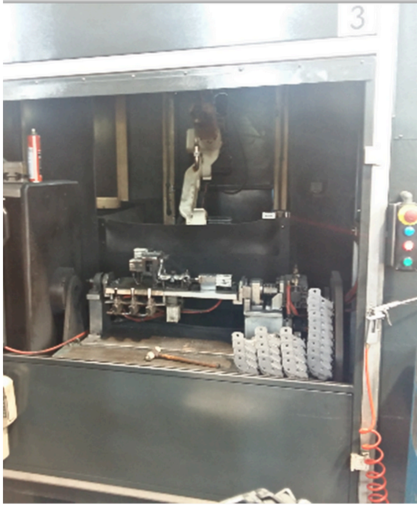
GAZ ALTI KAYNAK ROBOTO 350 A DAIHEN (1 Adet)
